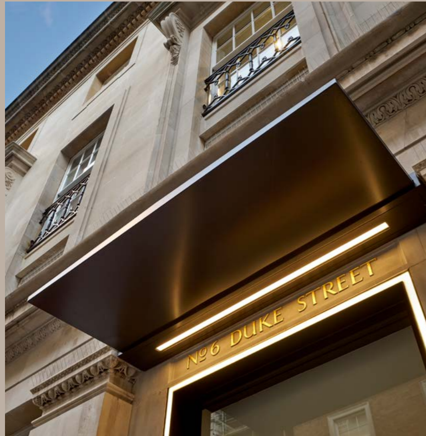
6 Duke Street St James's has been designed by Barr Gazetas to provide a contemporary yet classical St James's office building.
